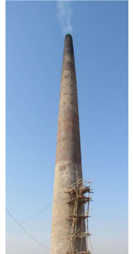
Invisible/light grey colour = Complete Combustion
