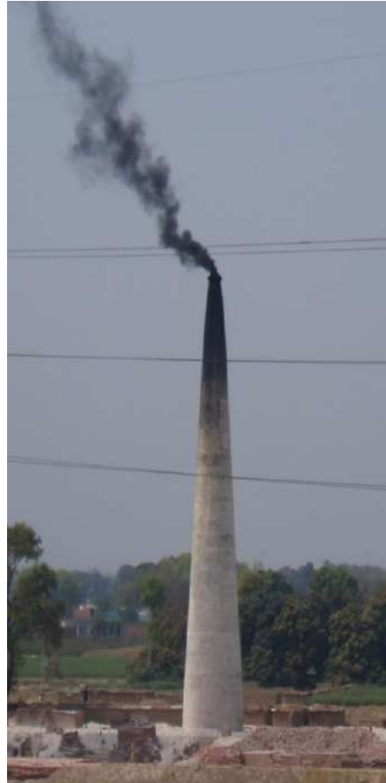
Black Smoke = Incomplete Combustion
