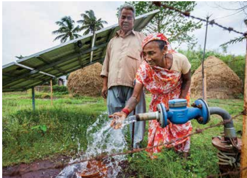
Irrigation using solar powered pumps in Saptari
