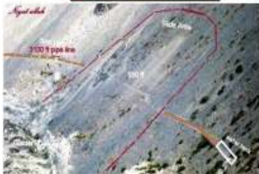
Rehabilitation of Gulkin Channel, Passu Glacier
