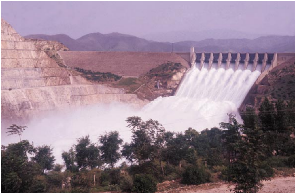
Mangla Dam (Source: WAPDA)
