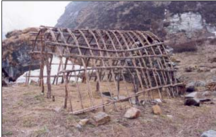
The bundles of bamboo together make a strong frame of ribs and girders. In the above 250cm high construction the side facing the strong winds is closed with a loosely piled stone wall, providing also stability to the construction.
