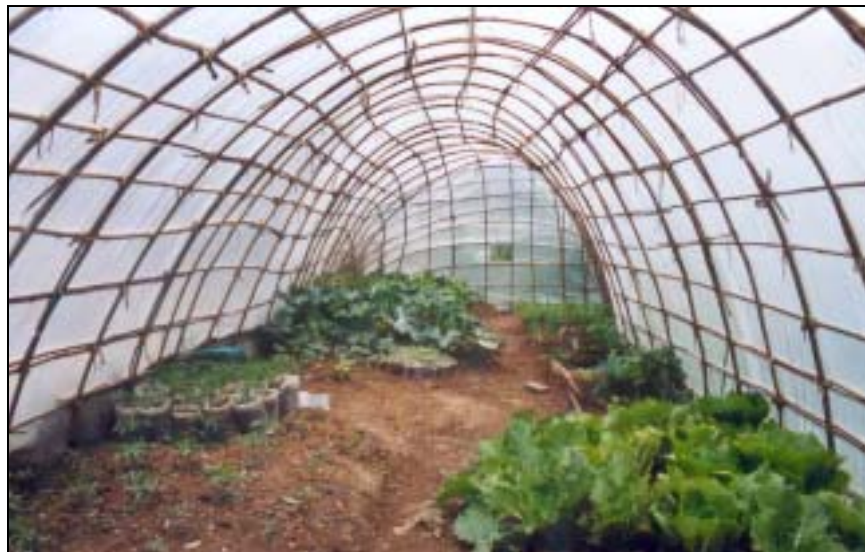
The bundles of bamboo together make a strong frame of ribs and girders. In the above 250cm high construction the side facing the strong winds is closed with a loosely piled stone wall, providing also stability to the construction.
