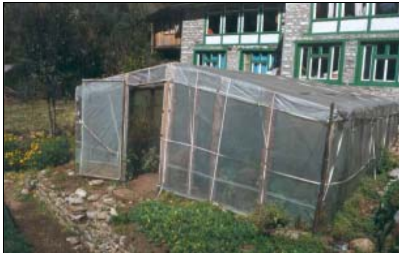
In this greenhouse in Pangdung, the foil is effectively tied down with packing straps nailed to the wooden structure.
