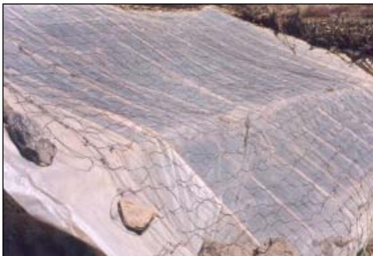
Without a strong bow frame rib construction and with improper fixing of the UV foil, the wind will rapidly damage the plastic foil.
