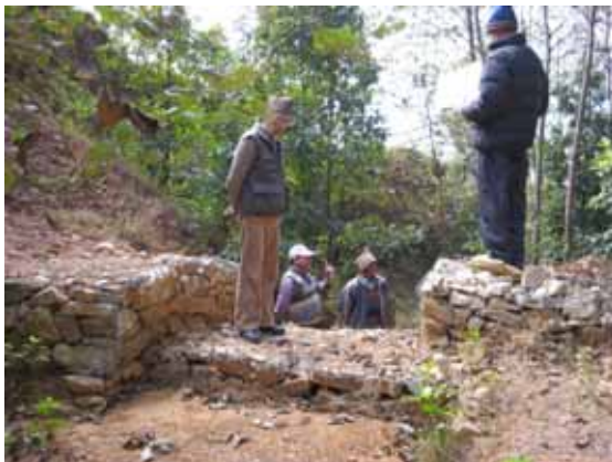
Photo 6. GCFUG members and DSCWM Technician observing check dam filled with sediment in one year
