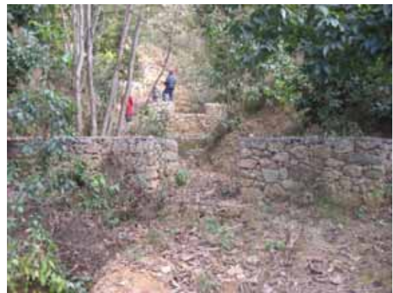
Photo 5. Series of small check dams
