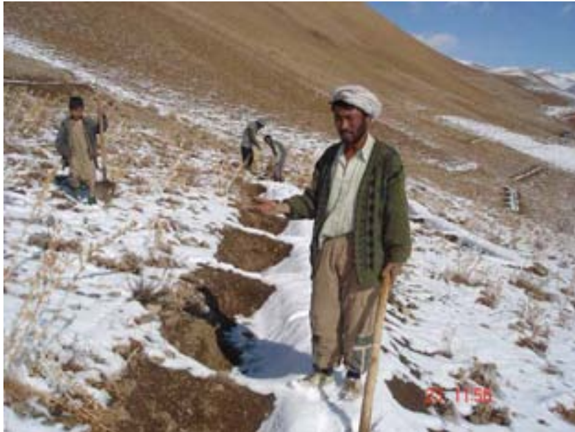
Picture: Compartmentalized and open trenches in Afghanistan (Andrew Billingsley)
