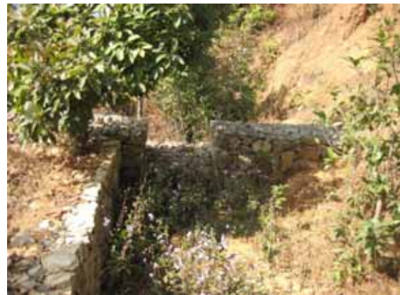
Photo 7. Check dam at outlet of gully from landslide area, filled with sediment in one year
