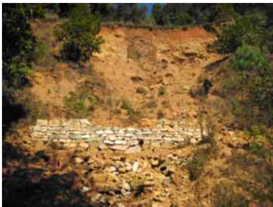
Photo 4. Loose stone retaining wall
