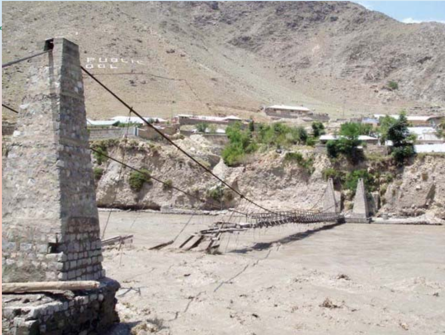
A suspension bridge over the Chitral River was destroyed by flash floods. PHOTO: APP
